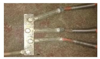
Closer inspection of the defective portable Primary HV earth found that the insulation and conductors were damaged under the sprung coil shrouds at another three positions. The earths were included in a formal inspection regime, and their next inspection due date was April 2016.
