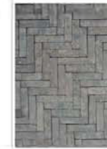
Clay Brick Paving - Highway
