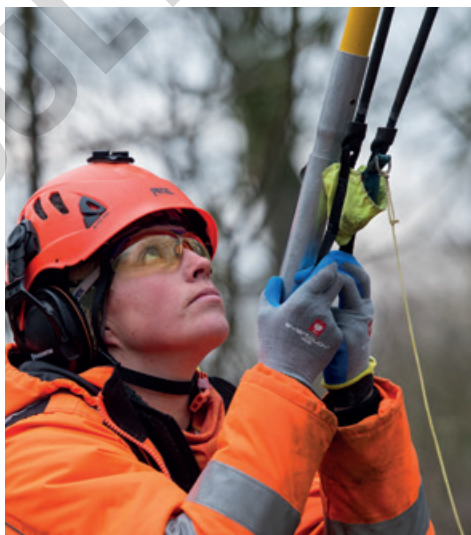
7.4.8 Using a catapult to achieve a greater throwline distance.
