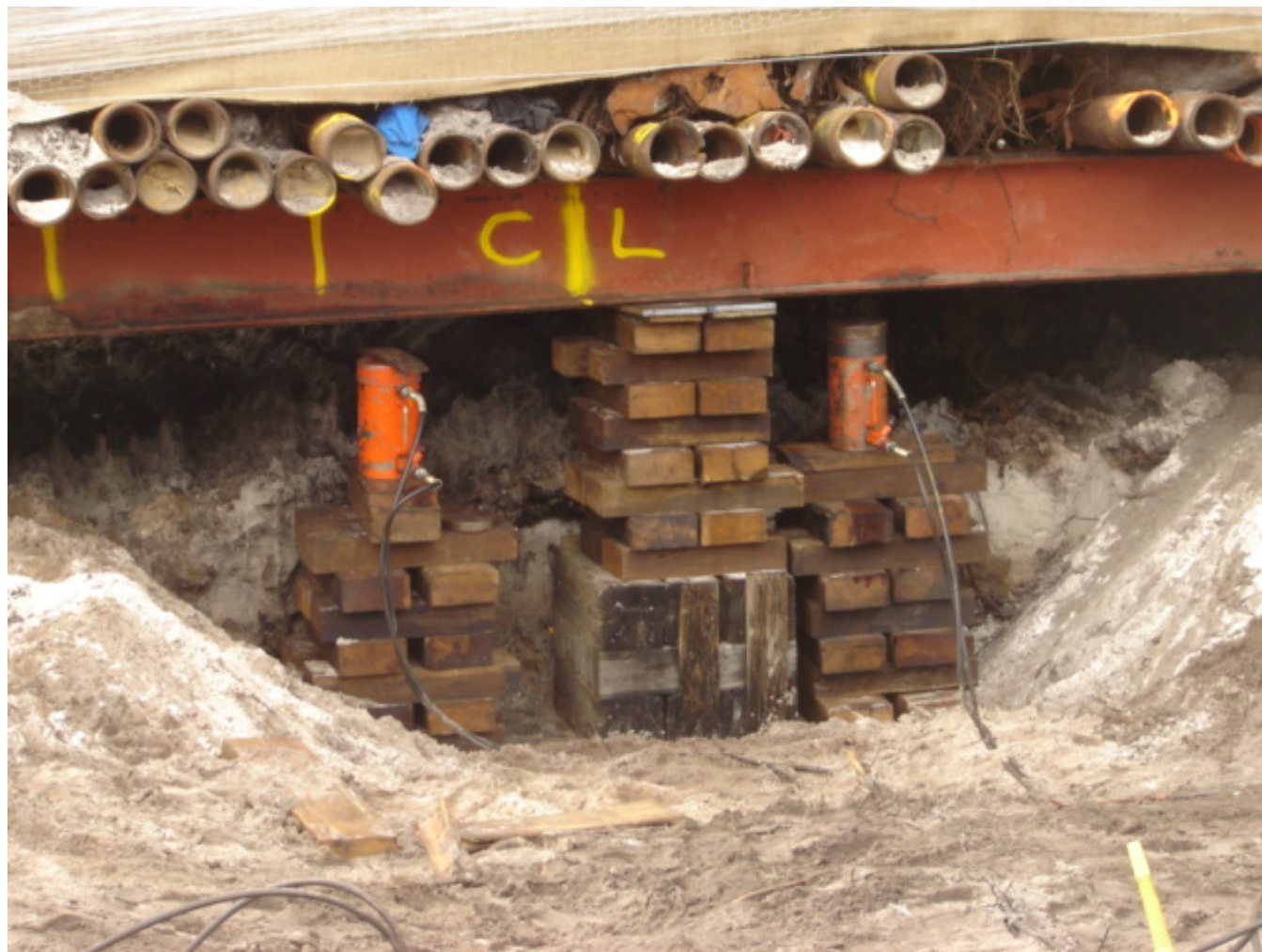
The Hollywell Fig – Ficus virens – Hydraulic jacks and cribs.
