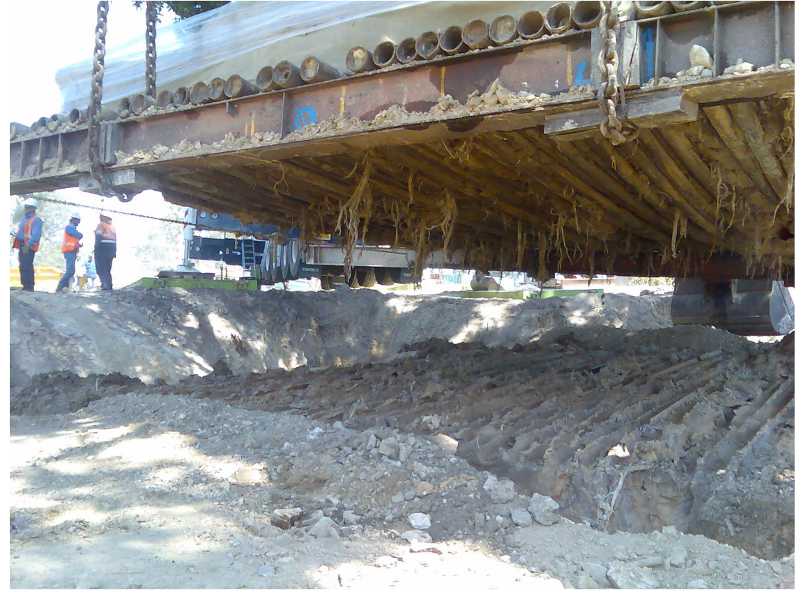
Crane lifted 160T fig with close spaced pipes to aid in root plate separation in heavy clay.
