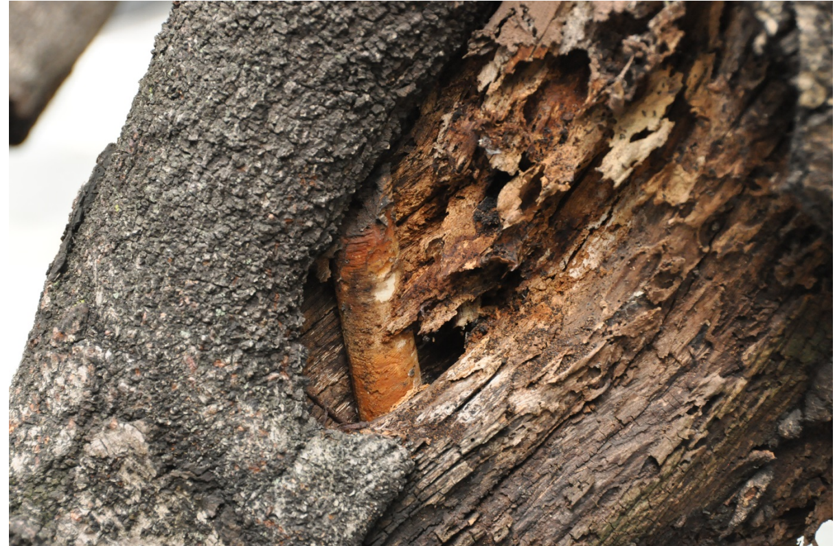
Wood decay with bolt hole filled with expansion foam.
