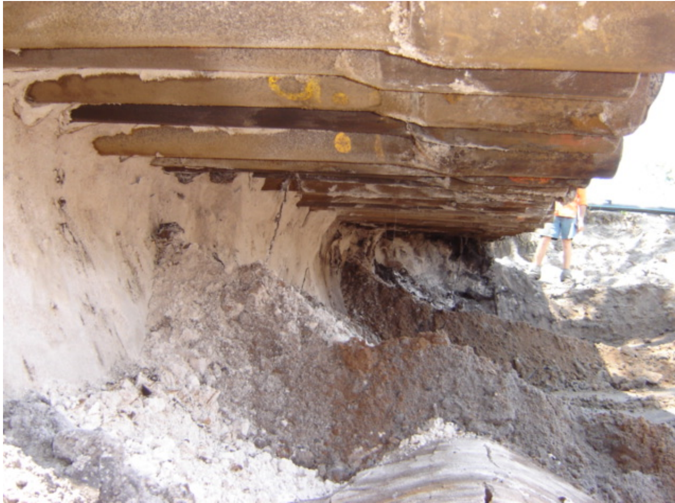
The Hollywell Fig – Ficus virens – Undercut for beam placement.
