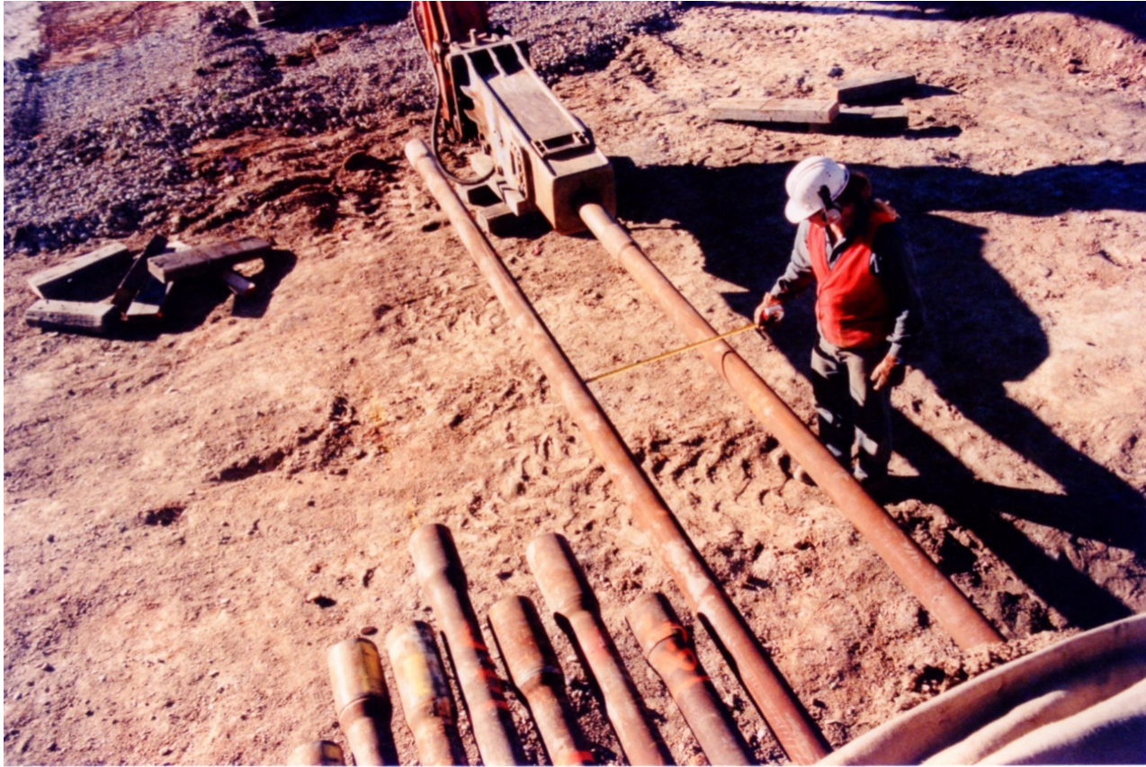
Pipe installation with rock hammer on 30T excavator.
