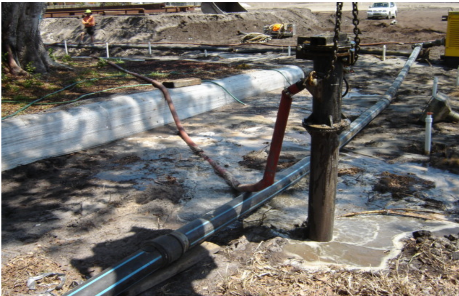
The Hollywell Fig – Ficus virens – Spear pump installation.
