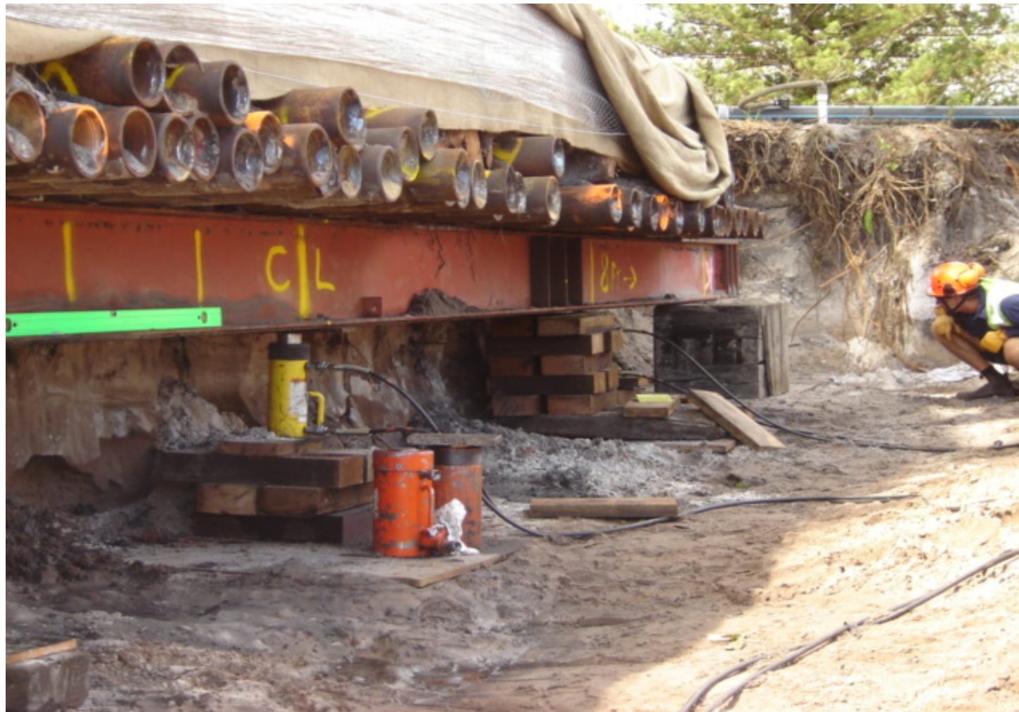
The Hollywell Fig – Ficus virens – Hydraulic jack installation.
