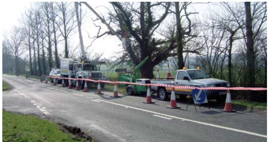
Team from AAAC Steve's Industries carrying out roadside work.
