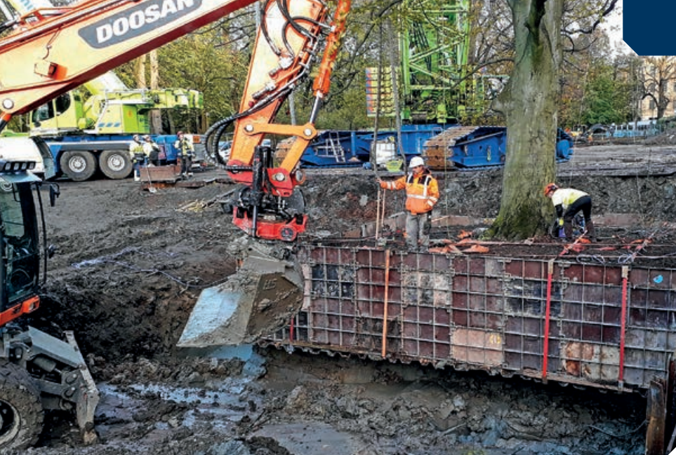
Figure 6: Heavy, saturated clay subsoil was just one of the challenges the project team faced in preparing the trees for lifting, but the combination of patience, skill, all the right tools and a real team effort meant that no problem was insurmountable. (Photo: Martin Gammie)
